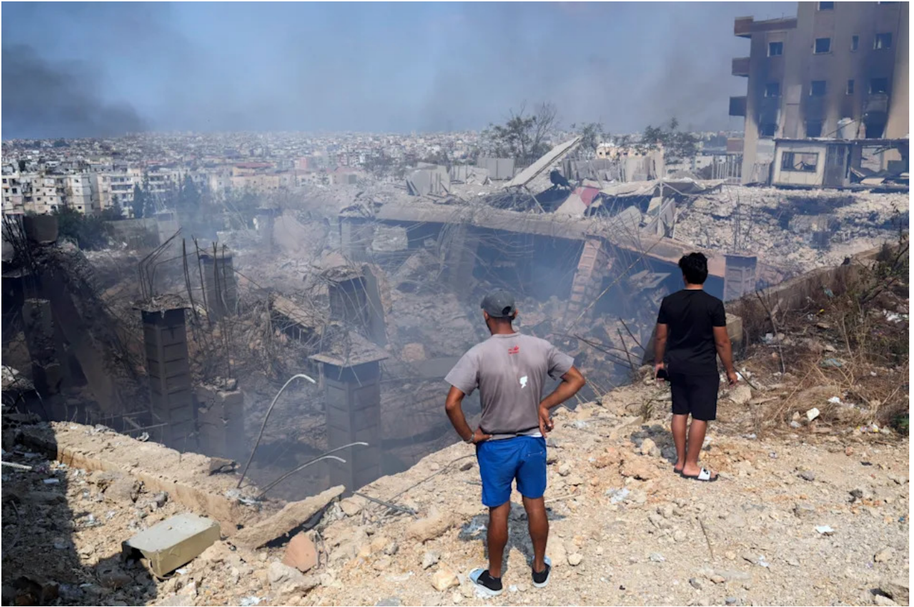
People check a damaged building at the site of an Israeli airstrike in Choueifat, south east of Beirut, Saturday, Sept. 28, 2024. (AP Photo/Hussein Malla)ASSOCIATED PRESS
